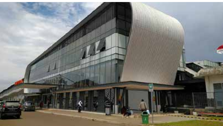
BSD City - Renovation of Cisauk Station
