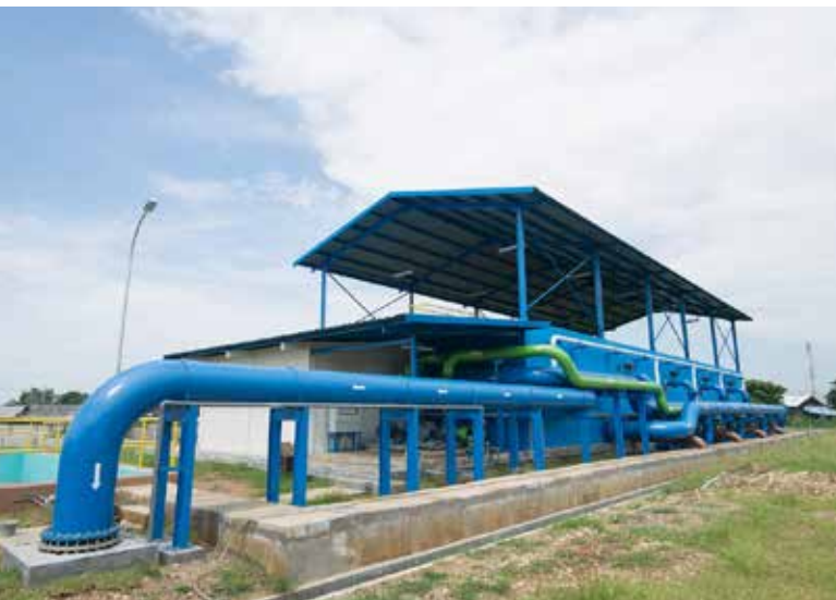
Industrial - GIIC - Water Treatment Plant
