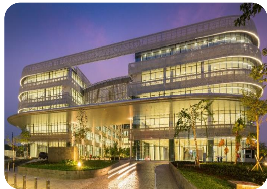
Green Office Park1 BSD
