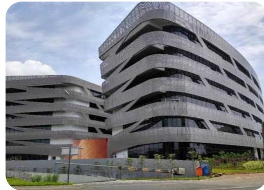
Green Office Park 9 BSD
