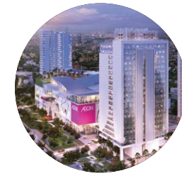
APARTMENT SOUTHGATE Jakarta
