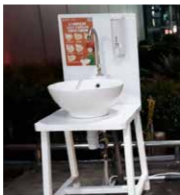
Penyediaan fasilitas portable handwash di ITC Depok Installation of portable hand wash facility at ITC Depok
